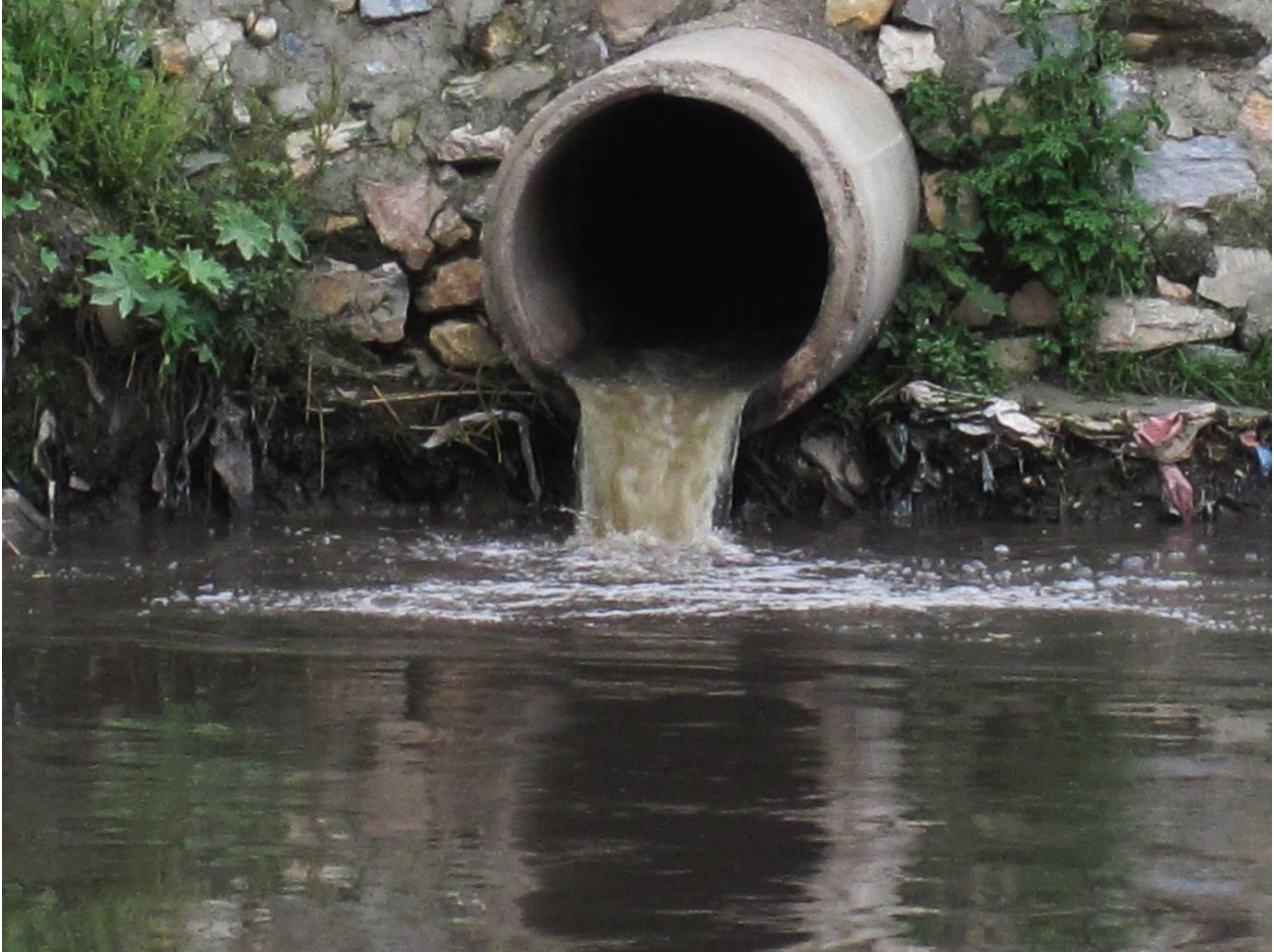
picture: Untreated sewage pours into the river
